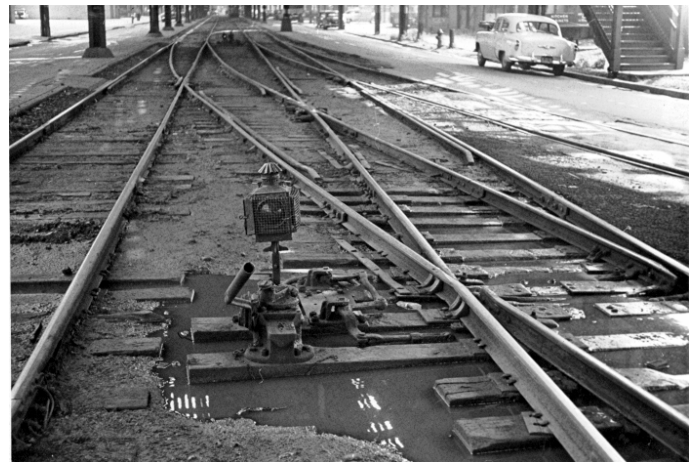
McDonald Avenue, south of Cortelyou Road, looking south, showing turnouts to South Brooklyn Railway, September 17, 1954.
