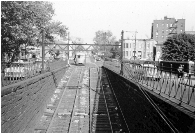
Two shots of the Ocean Parkway underpass on the Church Avenue Line, as it appeared on October 20, 1955. After trolley service ended, the tunnel was backfilled and the rails were donated to the Branford Trolley Museum, now known as the Shore Line Trolley Museum.
