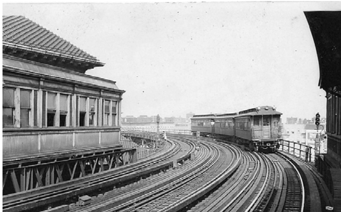
110 th Street looking north, June, 1940. Bernard Linder collection
