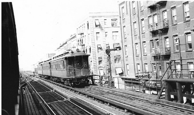
104 th Street looking north, June, 1940. Bernard Linder collection
