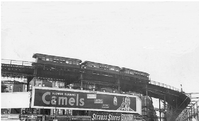
W. 110 th Street looking north, June, 1940. Bernard Linder collection
