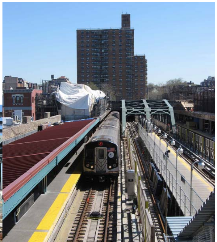
Alstom R-160A 9408 leads a northbound F train into Fourth Avenue station. View taken from the temporary overpass between the northbound platform and temporary southbound platform.
