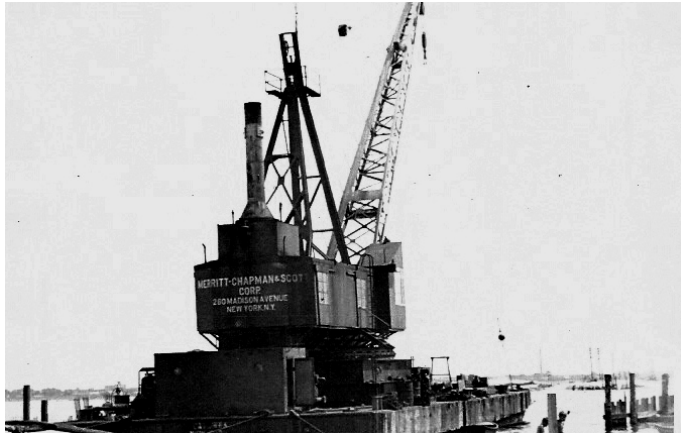
Pile construction at Broad Channel, August, 1954. Bernard Linder collection
