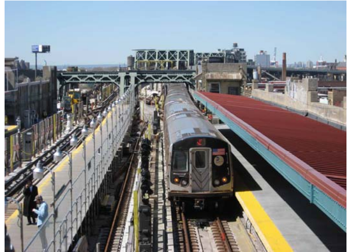
Looking west towards the Gowanus Canal bridge, we see a northbound ⑤ train composed of Alstom R-160As leaving the Fourth Avenue station.
