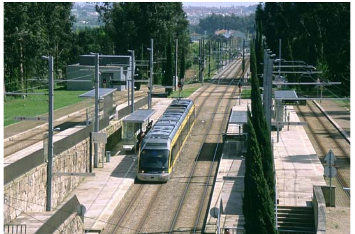
A view at the Verdes station. The Airport line uses the center tracks, which make a sharp turn from north to west under the B Line tracks.
