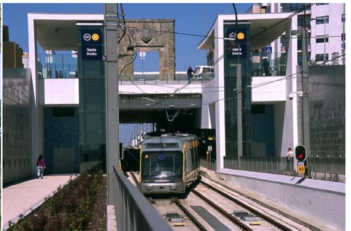
The southern end of the D Line is the Santo Ovidio station, where after discharging their passengers, trains pull up to just beyond the crossover and change ends. An area to store additional LRVs is behind the photographer. Elevators and escalators connect the platforms with a mezzanine and the street above.
