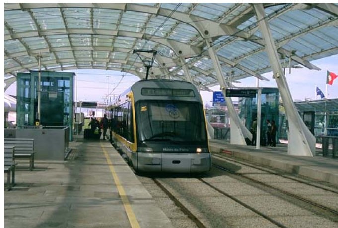
A Eurotram on the E Line at Porto's airport. This photo shows the escalators and elevators connecting the platforms to an underground corridor that leads directly to the arrival and departure lobbies.
