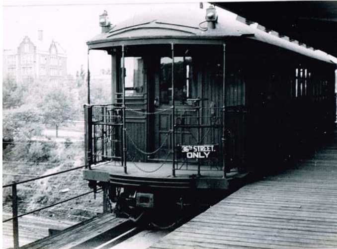
65 th Street station, Fifth Avenue "L," looking south. Bernard Linder collection
