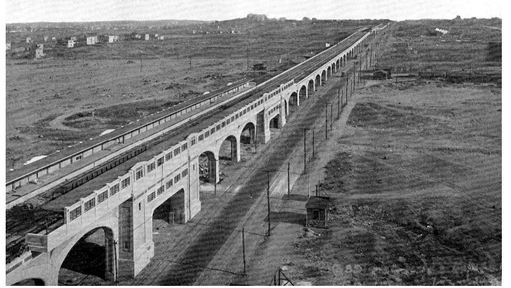
Birdseye view of Flushing Line reinforced concrete structure over Queens Boulevard.
