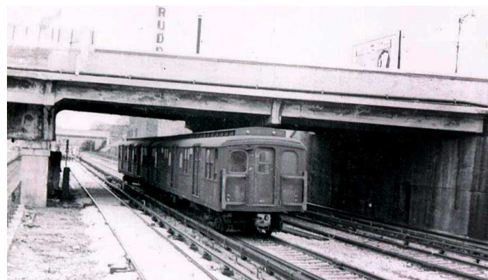
Looking west from 8th Avenue station. Bernard Linder collection
