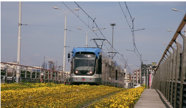
After leaving the street the inbound Bombardier car approaches the Mehmet Akif station in the center median of a short viaduct that had burst out in color. Goldenrods on the T1?
