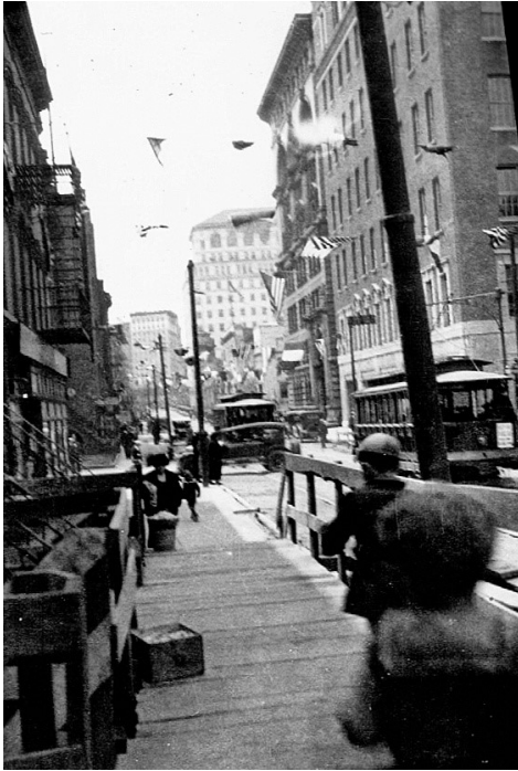
Willoughby Street near Lawrence Street, looking west, during station construction. Bernard Linder collection
