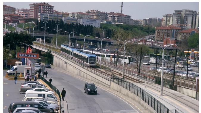
The outer portion of the T1 reaches the Zeytinburnu station, the original end of the line and a transfer point to the M1, via a long curving viaduct.
