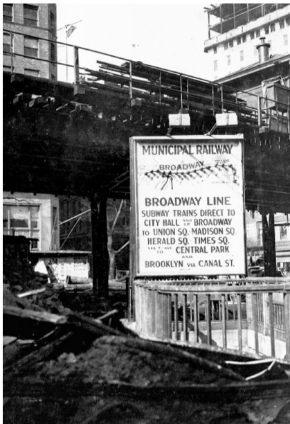
Whitehall Street station under construction. Bernard Linder collection
