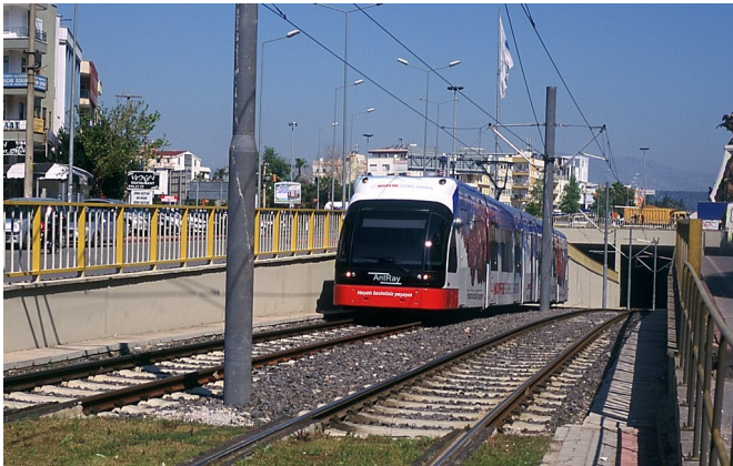
...with the Calli station located between the two ramps.
