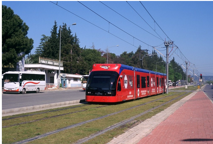
The northern end of the line is almost perfectly straight, and runs in the grassed-in center reservation of Antalya Blv. This view is near the Dokuma station.
