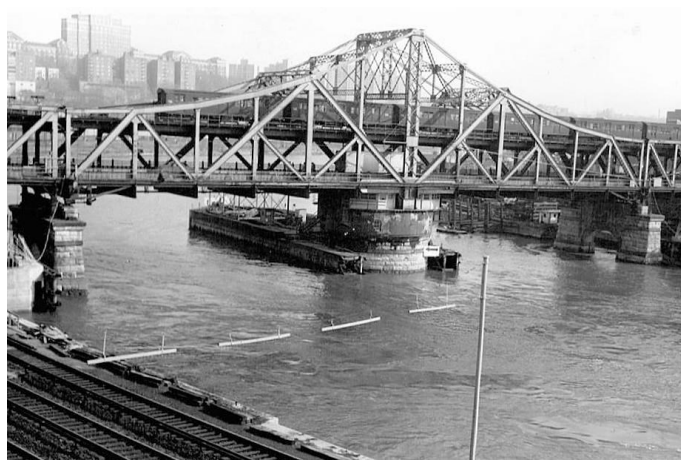
Second Broadway Bridge, looking east, April 25, 1959. Bernard Linder photograph
