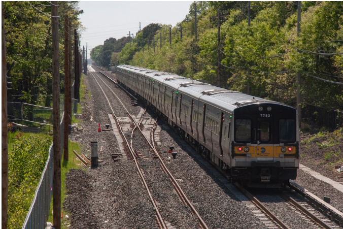
Train #2057 heading west through the future Danch Interlocking on May 21, 2018. The second track still lacks third rail and none of the four new signals have been installed yet.
