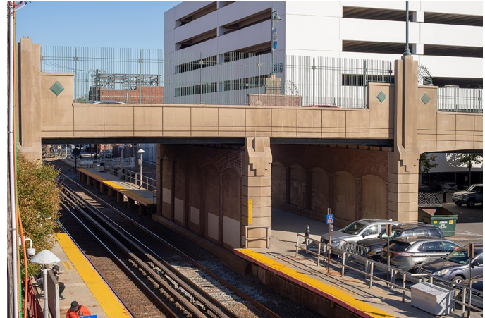
When the Mineola Boulevard bridge was reconstructed several years ago, provision was made for the future third track, shown here on the right side of the center abutment. It is not clear to me whether there will be sufficient space for an island platform where the existing eastbound platform is so that Mineola can be an express stop. Mineola is, after all, the seat of Nassau County government. Photo taken on October 25, 2018.
