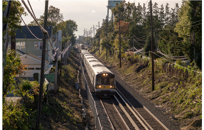
Looking west from the Ellison Avenue overpass in Westbury towards the Carle Place station on November 6, 2018 we see M-7 7818 (Bombardier Transportation, 3/2007) leading train #1714 from Penn Station to Huntington. You can see just how close the right-of-way is to the houses on the south side of the right-of-way here. From east of Mineola station to a point between here and Westbury station, the new third track is supposed to be on the north side of the right of way, to the right in this photo. Roughly five miles of new retaining and sound barrier walls will need to be constructed along the project corridor.
