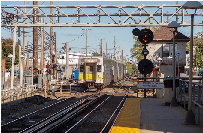
C-3 5001 (Kawasaki Railcar, 12/1998) leads train #651 from Port Jefferson to Long Island City into Mineola at 2:36 PM on October 25, 2018. Nassau Tower, just beyond the eastbound platform here, will need to be demolished to make way for the third track. All of the interlockings in the project area will be controlled from the Jamaica Central Control building with backup from the existing Queens and Divide Towers. The Main Street crossing, under the rear end of the first car, will either be completely closed to traffic and be replaced with a pedestrian bridge (the preferred alternative) or it may become a one-way northbound underpass (also with a pedestrian bridge) while Willis Avenue, just beyond the locomotive on the rear of the train, will be converted to an underpass. That little grade crossing right in front of the train is a pedestrian crossing, which will also be closed.
