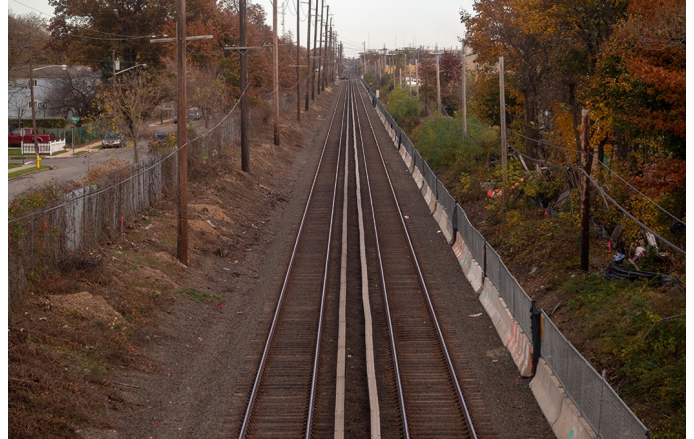
Looking east from the Grand Boulevard overpass in the hamlet of New Cassel on November 7, 2018. This is between the Westbury and Hicksville stations. Some where in this view all three tracks will take a very slight jog to the north (to the left in this view) and the new third track will be on the north side of the right of way from here. In the distance is the easternmost grade crossing of this project, Urban Avenue. It, too, will be replaced by an underpass.
