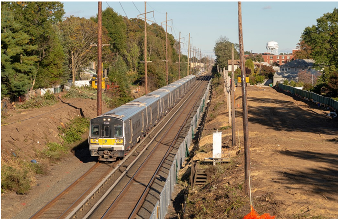
M-7 7305 (Bombardier Transportation, 10/2004) leads train #1709 from Huntington to Penn Station just east of Ellison Avenue in Westbury on October 25, 2018. It is not known to me why the large area to the right, or the smaller area to the left, have been cleared. I had thought that this was going to be for a new traction power substation but I have learned that the existing substations will all be rebuilt in place, as had been done at Substation G13 in Floral Park in 2010. In this view the current two main tracks are to be shifted slightly south (to the right) and the new third track is supposed to be on the north (left) side. Between here and Post Avenue in Westbury in the distance, all three tracks need to shift south again as the new third track is on the south side of the right of way through Westbury. All of these track shifts will be engineered for 80 MPH maximum speeds.
