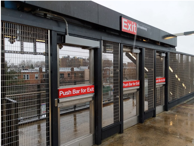
At Broadway N W , which reopened on 1/24/2019, an entirely new exit staircase was built towards the south end of the northbound platform. This will help to reduce the volume of passengers exiting through the fare control area on the mezzanine.
