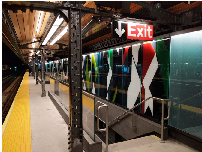
Looking down one of the platforms at 39 Av-Dutch Kills N W on 1/28/2019, opening day. Almost everything in this view, save the original ironwork, is new: platform walls, railings, lighting, platform surface, canopy, and lighting.
