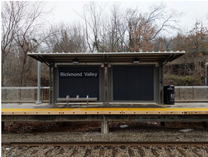
A view of the shelter shed in the center of the eastbound platform at the Richmond Valley station on the Staten Island Railway. This station, along with 34 St-Penn Station (A C E), was not closed during its renovation.
