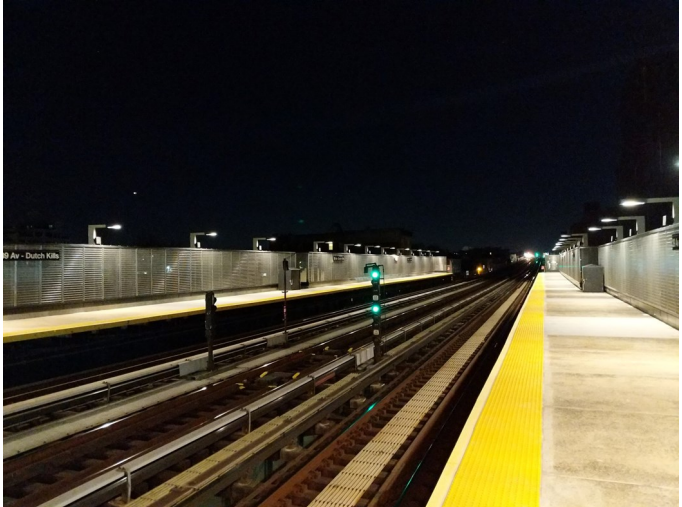
Looking north on the northbound platform, the new LED lighting is very evident and also has a pleasing color temperature. The corrugated metal walls were replaced with a stainless-steel mesh. Providing less shelter from the wind, especially in winter, it does create a more open environment as you can now see the streetscape below.
