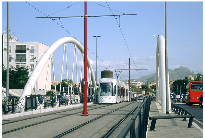
The construction of a new arched bridge over the Oreto River for Corso dei Mille was part of the project to build Route 1 of Palermo's new tramway. This is a view looking eastward showing an inbound car.
