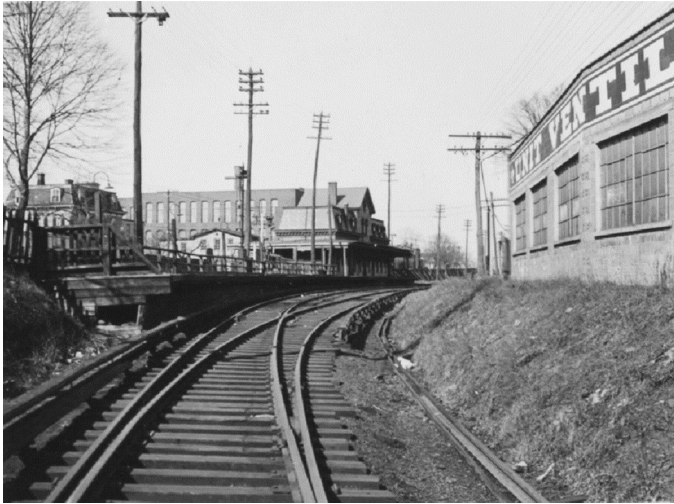
View north at the College Point station, 3/3/1932. The entire branch was single-track with passing sidings here at College Point and at Flushing-Bridge Street and Whitestone.
