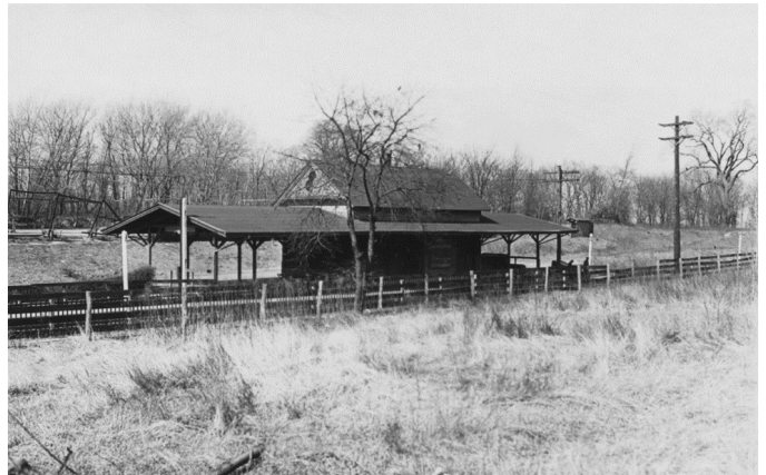
View northwest of the Whitestone Landing station, 3/5/1932.
