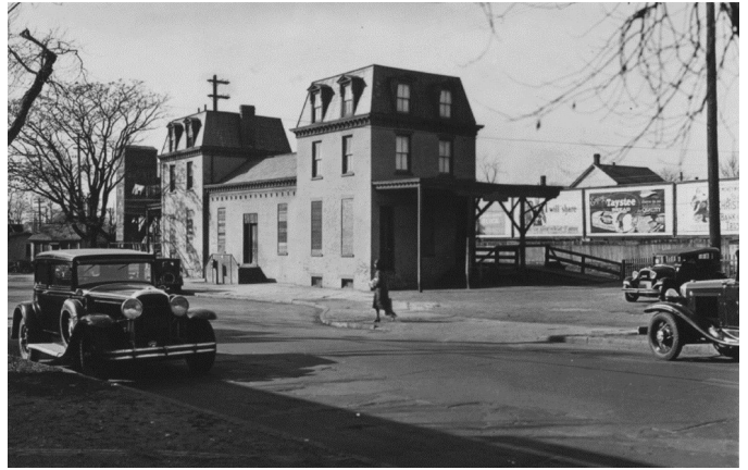
Looking northwest at the Whitestone station, 3/5/1932. This street (15th Avenue at the time) is now the eastbound service road of the Cross Island Parkway. The parkway, in a depressed cut here, is on the railroad right-of-way.
