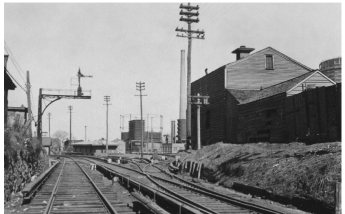
View north from a little east (railroad direction) of the Flushing-Bridge Street station. The tracks to the right lead to the Flushing-Bridge Street team yard, for freight cars. The manual block signal for clearance to College Point is overhead. 3/3/1932
