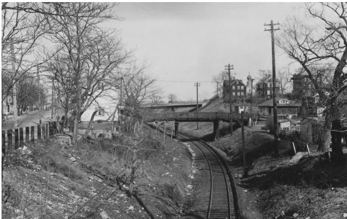
Looking east from east of the Whitestone station, we see the 150th Place and, beyond it in the distance, the Cross Island Boulevard (today's Clintonville Street) bridges. The 150th Place bridge may be from 1869 when the Flushing & North Side Railroad built the line. The Cross Island Boulevard bridge, like the Malba Drive bridge above, was built in 1908 and is the only other concrete bridge. 3/5/1932
