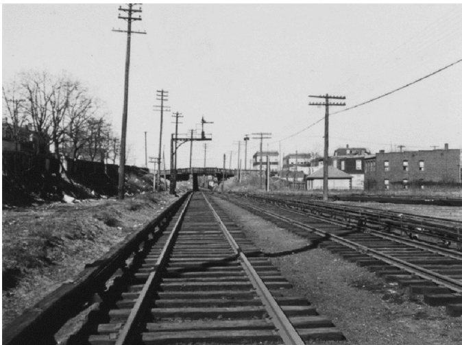
Looking north from just off the end of the platform at the College Point station, we see the next manual block signal, which gave clearance to the end of the line at Whitestone Landing; 3/13/1932.
