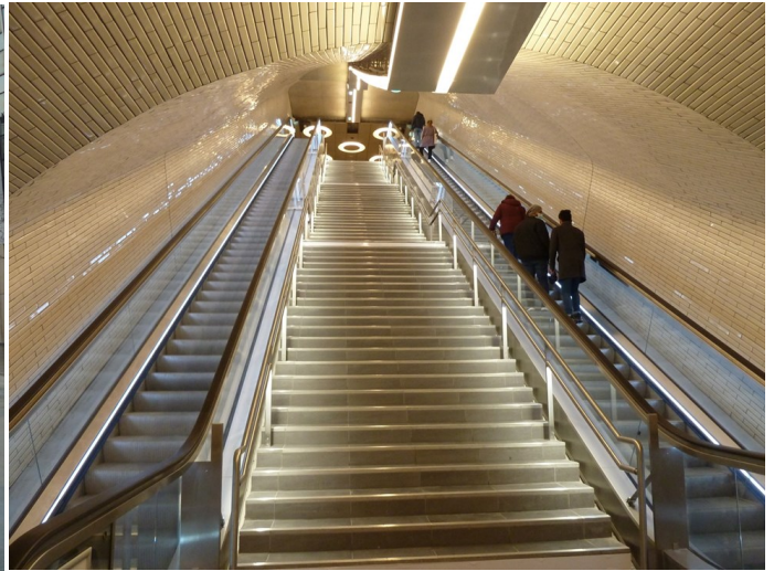
The depth of the Porte de Clichy station is clearly apparent in this view of the escalator shaft between the lower and upper mezzanines.
