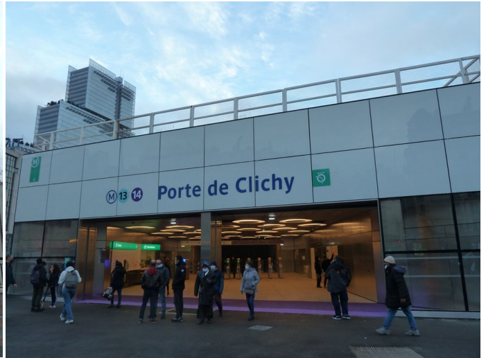
A head-on view of the new primary entrance headhouse at the Porte de Clichy station on January 28, 2021.
