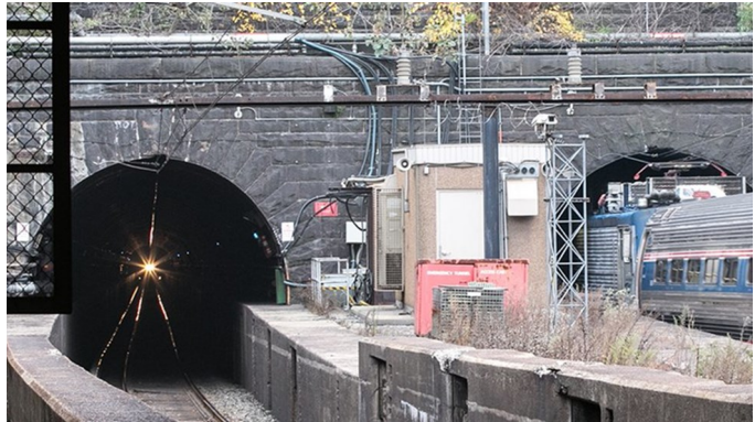
The New Jersey end of the Hudson River Tunnels. Amtrak photograph
