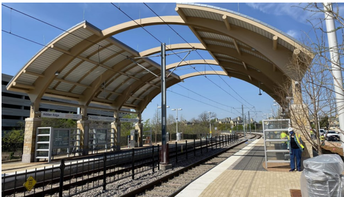
DART's new Hidden Ridge station on the Orange Line. DART photograph
