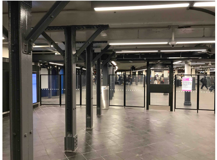
Looking southeast from the free zone towards the shuttle platform. The columns on the left used to be between Tracks 2 (left) and 1 (right). Subutay Musluoglu photo
