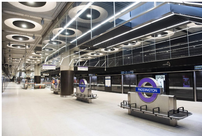
Paddington station on the Elizabeth Line. Transport for London photo
