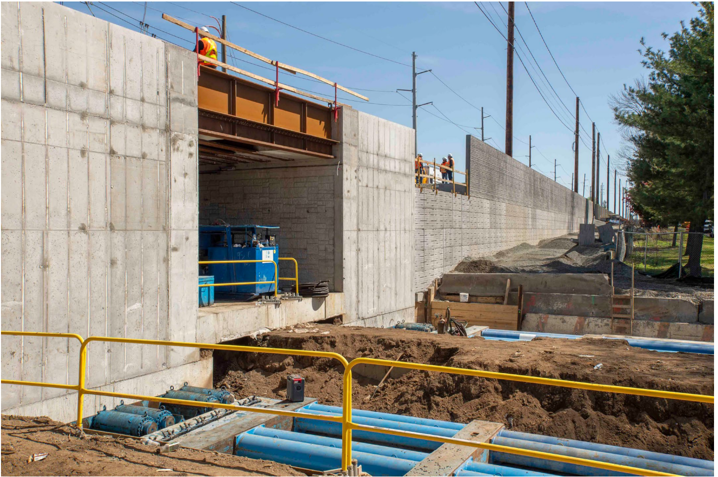
(Above) The view from street level, looking northeast. The box jacks are in blue in the ground. Jeff Erlitz photo
