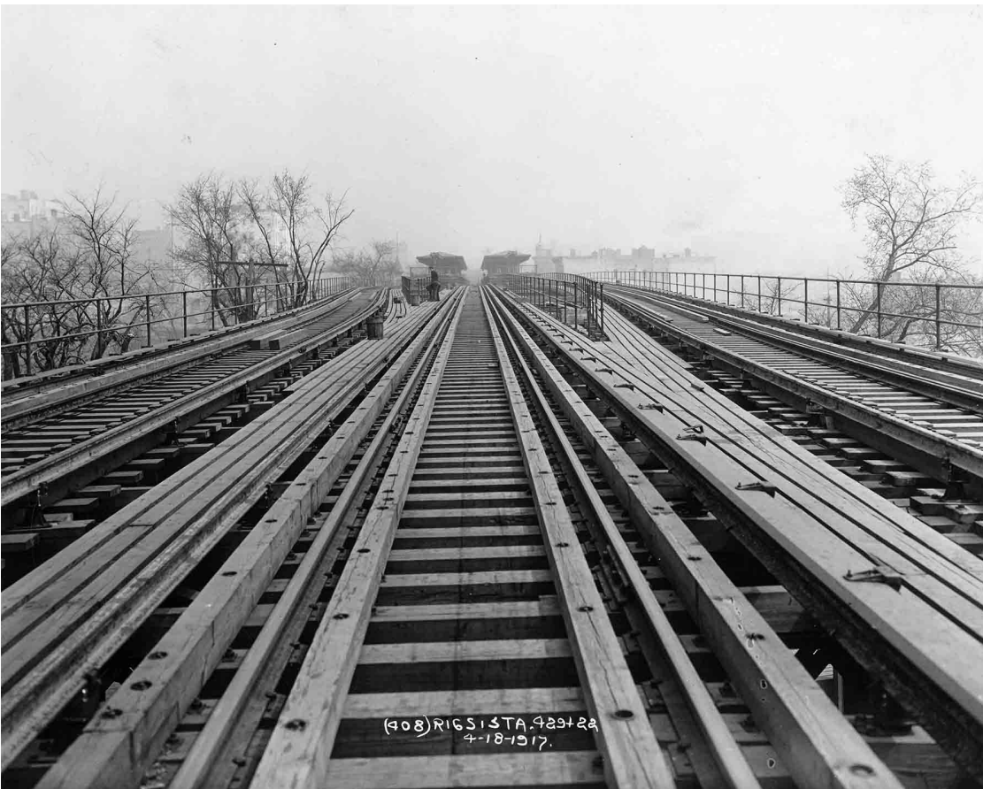
View north (actually northeast) south of New York University [Burnside Avenue] Station. Note that there are no crossover switches between the southbound local Track 1 and the middle Track M. This was the situation here until 1929. In that year, one crossover was installed here and one north of the station. The switches (and presumably the signals protecting them) were operated by "ground" levers on the walkways. In early 1930, an 11-lever US&S Style EP interlocking machine was installed at the north end of the northbound platform to control the two crossovers and the six home signals. By May of 1932, an actual tower was constructed just north of the platform, with a 19-lever US&S Model 14 machine. Pierre P. Pullis/PSC photo
