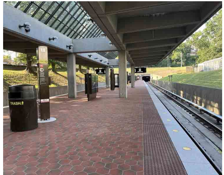
Updated Grosvenor-Strathmore platform with new non-slip tiles, a refurbished granite edge and new passenger information displays. WMATA photo
