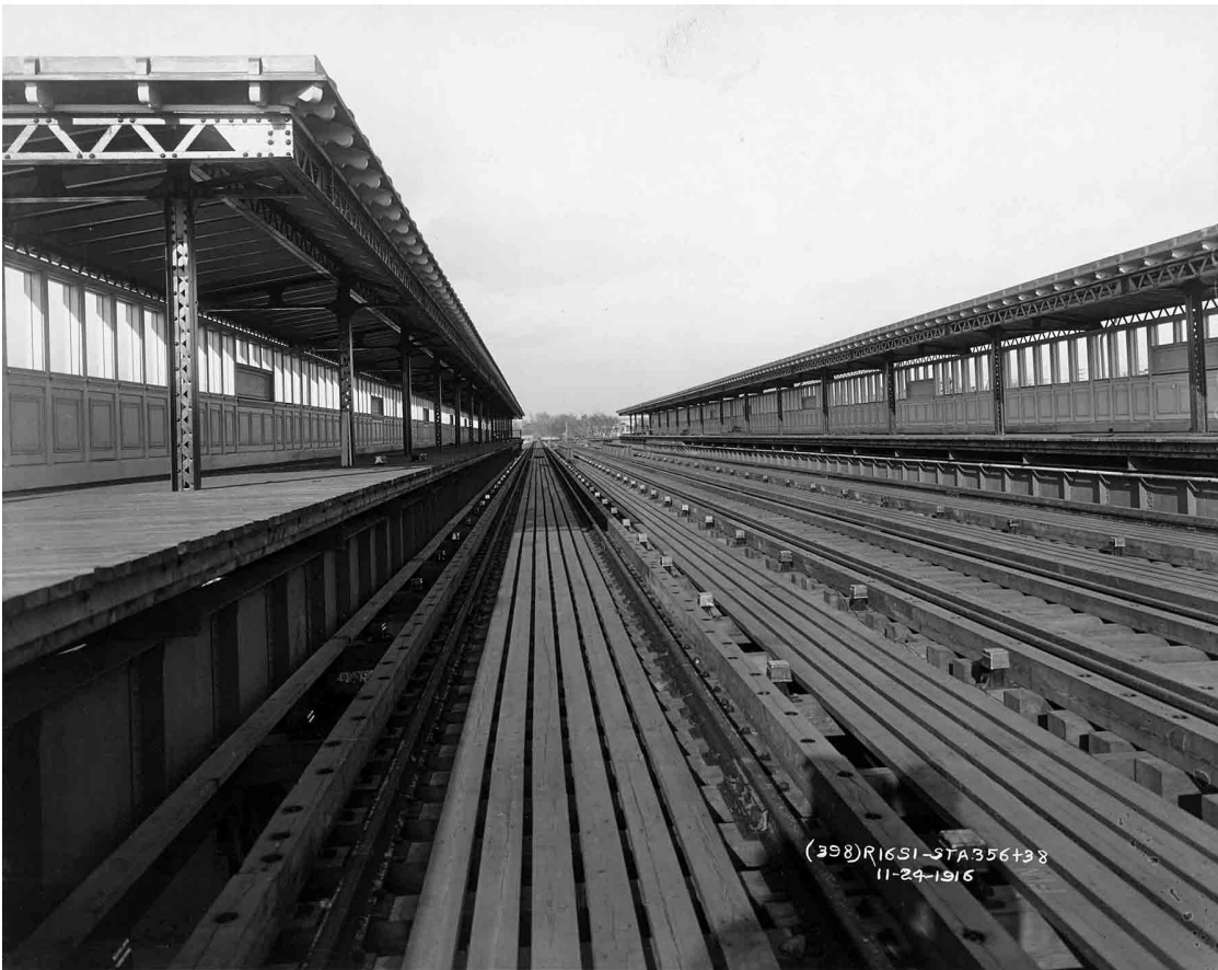
Still November 24, looking north up the southbound local Track 1. Note that since this is north of the junction with the Ninth Avenue Elevated, there are third rail insulators/supports for both subway type and elevated type third rails.
