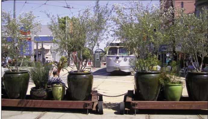
Steel gates with planters block off the plaza at 17th Street. On the rare occasions when the ramps at the Eureka Valley station (pg. 27) need to be accessed the gates can be rolled open.
