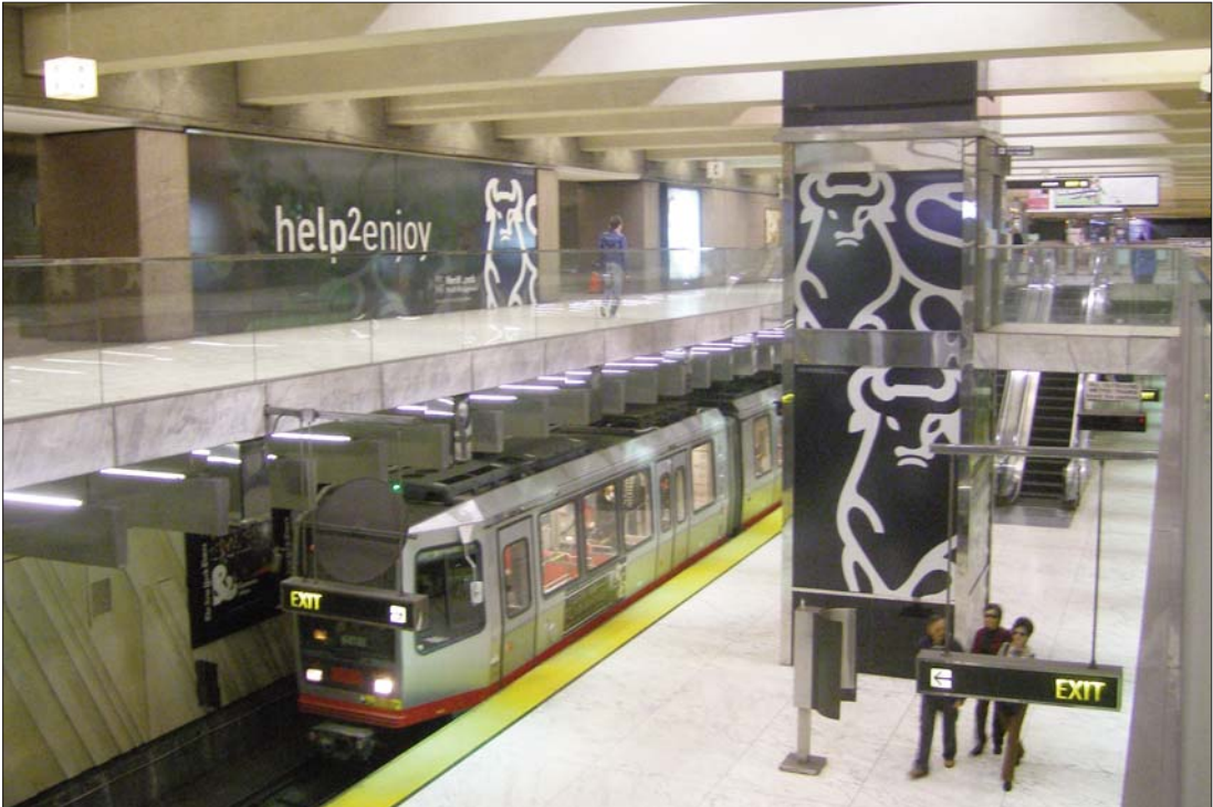
View of the Muni Metro platform from the galleries on the mezzanine. The elevator to the platform is at the center right of the photograph. A bridge leads from the mezzanine to the elevator. All underground stations on the Muni Metro are wheelchair accessible.
